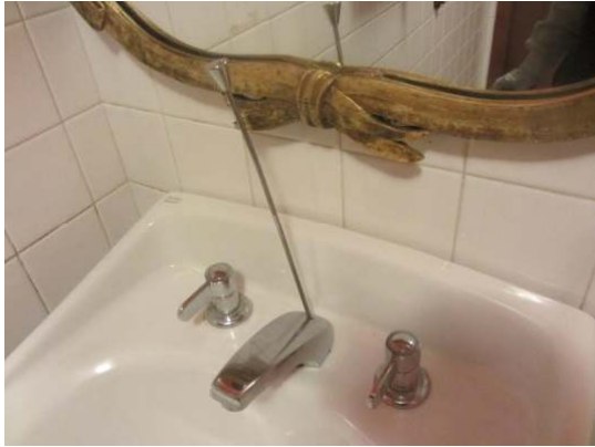
Ladies room drain stop not functional and entry door out of alignment
