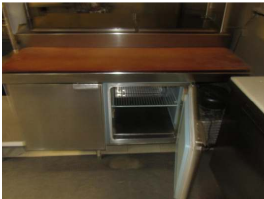
Cooling drawers under line not functional at the time of the inspection
