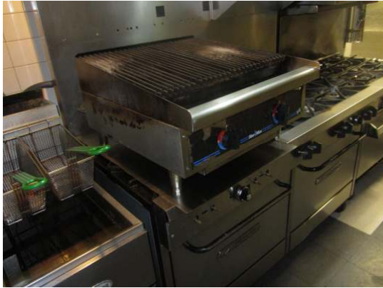
Portion of range burners not function. Fryer internals, suggest service and general maintenance on kitchen equipment due to age
