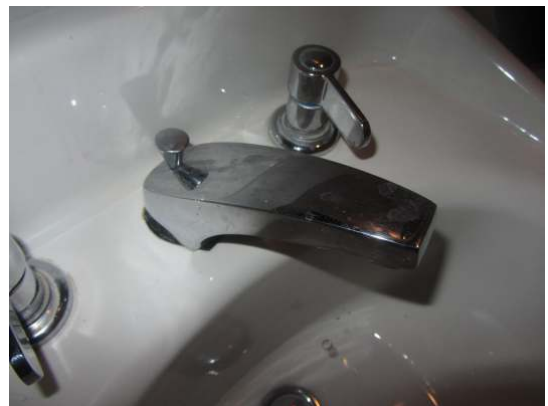
Kitchen restroom sink loose at the wall and faucet handles improperly fixed
