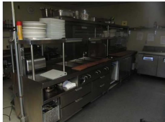
Cooling drawers under line not functional at the time of the inspection
