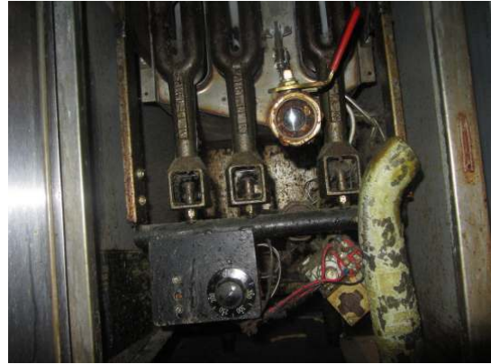
Portion of range burners not function. Fryer internals, suggest service and general maintenance on kitchen equipment due to age
