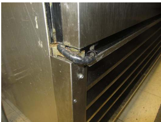
Wall freezer wiring field repair noted
