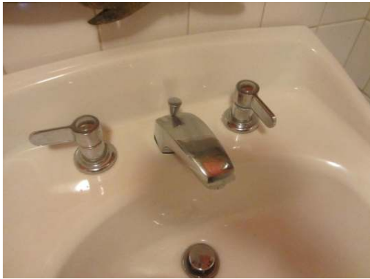
Mens room faucet handles improperly fixed and toilet continues to run water
