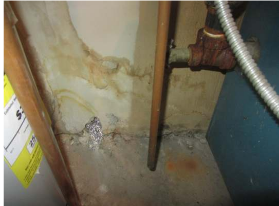
Active water leak at water heater union with water damaged walls noted
