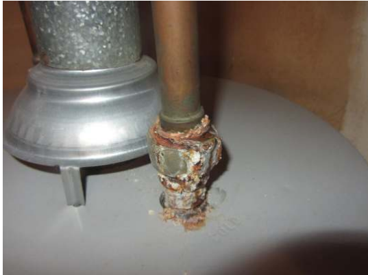
Active water leak at water heater union with water damaged walls noted
