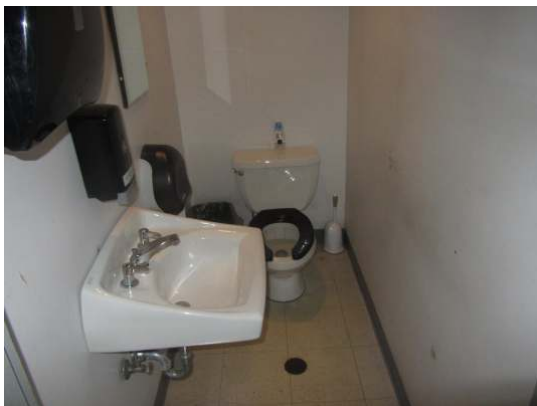
Kitchen restroom sink loose at the wall and faucet handles improperly fixed
